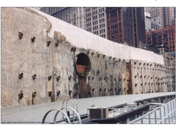
View showing remaining portion of the south tube, visible in the east slurry wall
